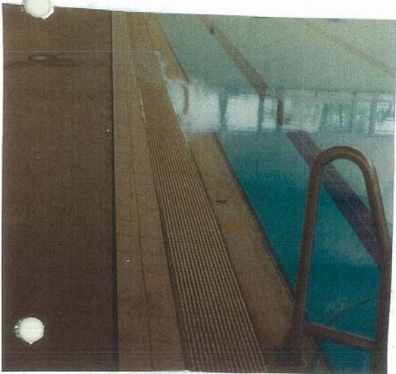
Typical Level Deck T With patient chair lift Level or Wet deck sic
