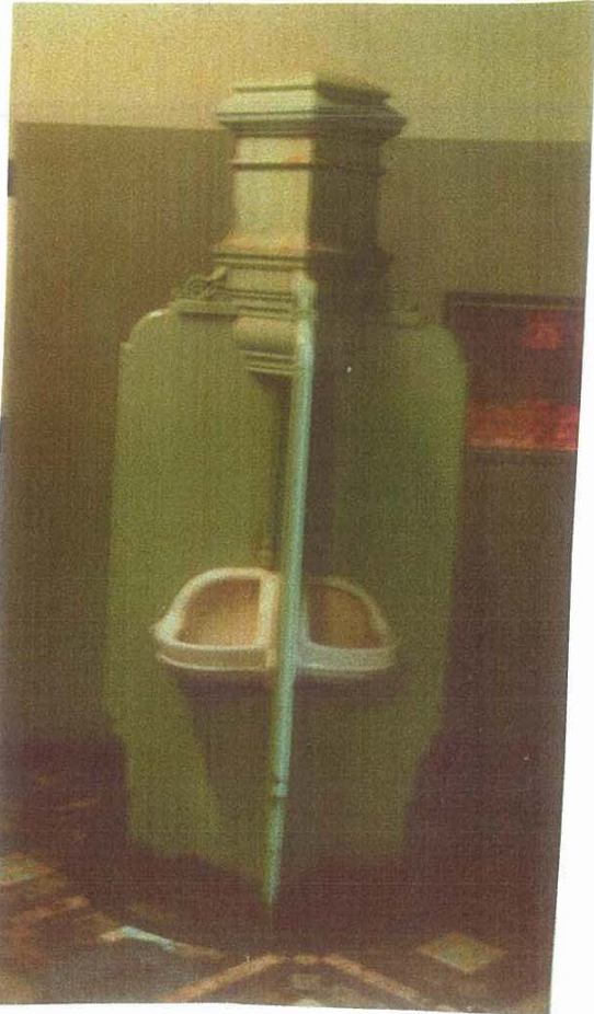
This Information included for historic interest only. Both the Burlington bell Water waste prevention cistern and the four way island Urinal with and floor grating was photographed in the Queen Victoria Building at Town Hall prior to the they were preserved.
